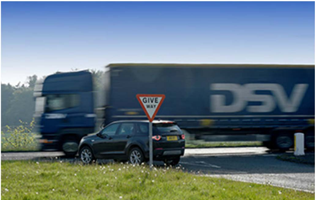
Image 5 – Existing Junction at Charlton Mires
