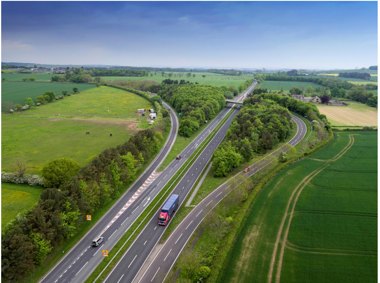
Image 3 – Existing Junction at Warreners House
